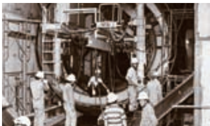
1977年地鐵隧道內壁被吊至適當位置。 Lifting of MTR tunnel linings into place in 1977.
