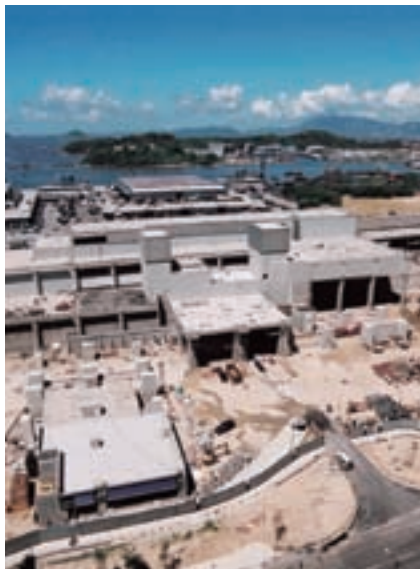
興建中的西鐵南昌站。 West Rail's Nam Cheong Station under construction.
