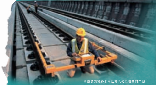
西鐵高架鐵路上用以減低火車嘈音的浮動路軌結構。 Floating track structure used on West Rail viaduct to reduce noise from trains.
