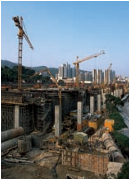
興建中的馬鞍山鐵路車公廟站。 Construction of Che Kung Temple Station on Ma On Shan Rail.
