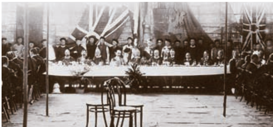
1909年廣九鐵路（華段）的廣州總站奠基，當局設宴慶祝。 Banquet held in 1909 to celebrate the laying of the foundation stone for the Canton Terminus of the Chinese Section.
