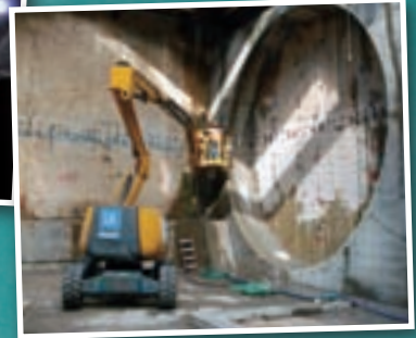
車站挖掘工程後可見未打通隧道的末端。隧道鑽挖機打通隧道後，便能與車站月台連接。 End face of tunnel after station excavation before tunnel boring machine breaks through to connect the station.
