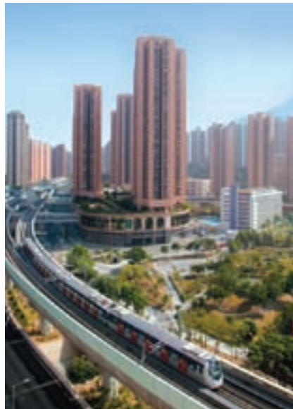
列車由馬鞍山站開出。 Train leaving Ma On Shan Station.
