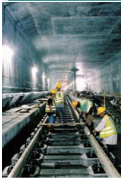
柯士甸站主路軌旁用以停泊回廠火車的存車軌道。 Pocket track next to the main track at Austin Station to park out-of-service trains.
