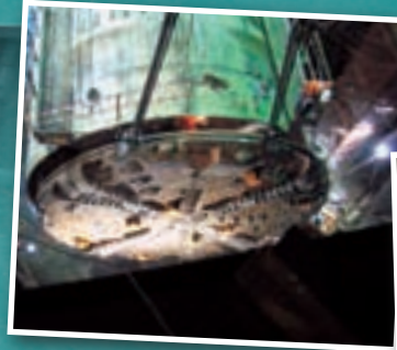
用以鑽挖隧道的鑽挖機的切剖面，擲於鑽挖機放置就緒，以便進行鑽挖隧道前。 Cutting face of tunnel boring machine being lowered into place before commencing tunnel boring.
