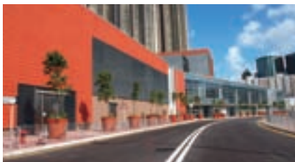
九龍南線的柯士甸站。 Austin Station on the Kowloon Southern Link.
