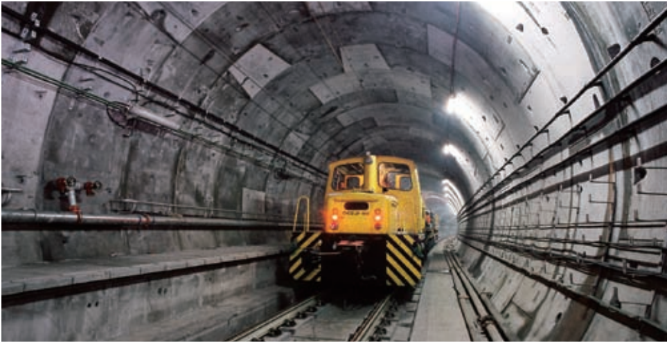
The KSL is on track for commissioning in the second half of 2009
