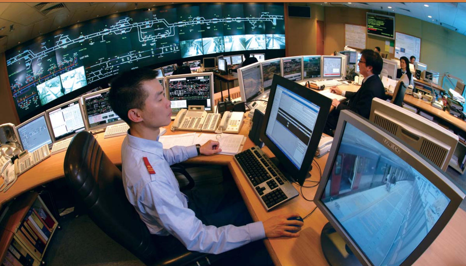
The East Rail Control Centre manages all traffic on East Rail and Ma On Shan Rail.
